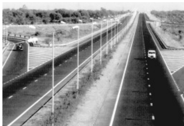
Fig.7.2: Ahmedabad- Vadodara Expressway
