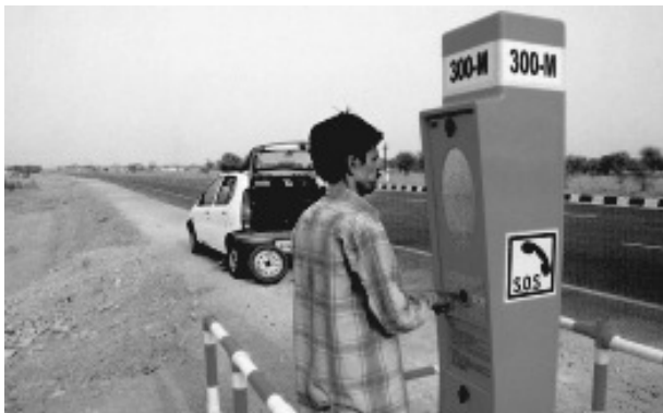
Fig.7.10 : Emergency call box on NH-8
