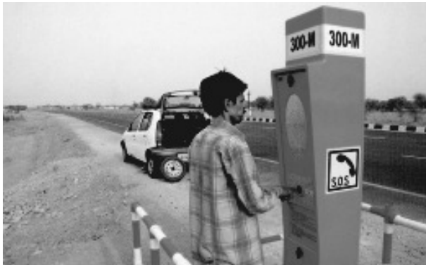
Fig.7.10 : Emergency call box on NH-8
